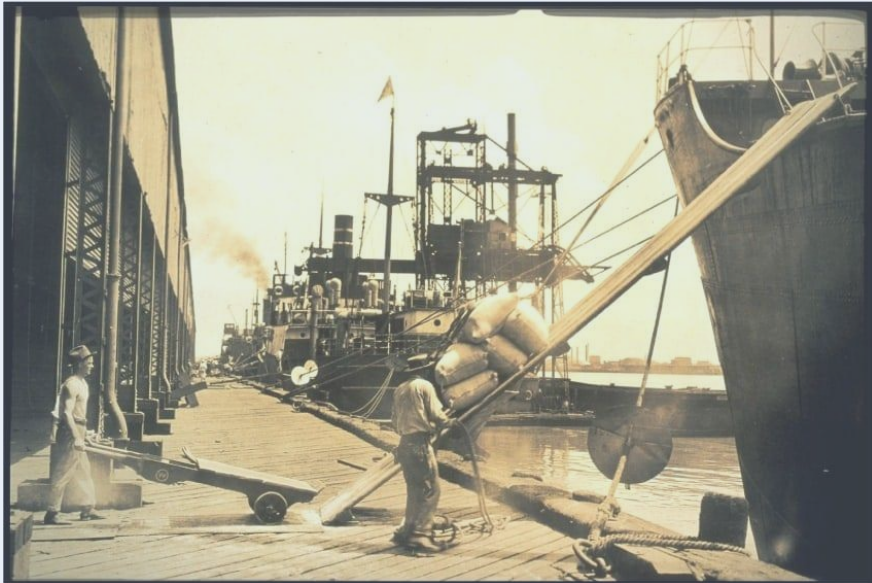
Loading break-bulk cargo at the Port of New Orleans, early 20th century. Source: Port of New Orleans (historical photograph), Public Domain .
